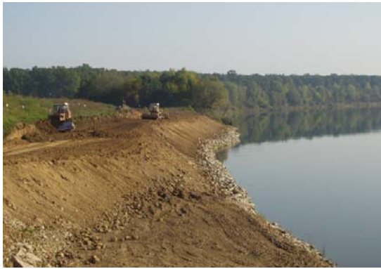
Figure 3.6a Bank protection under construction
